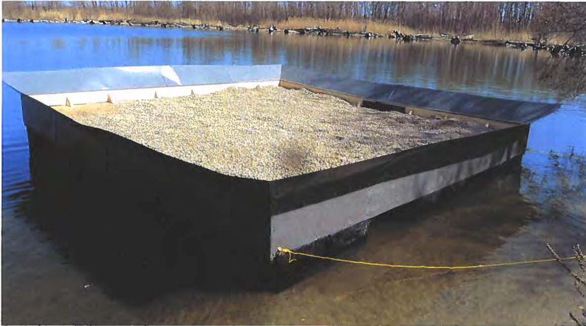
Completed platform at Lake Erie with predator guards, and pea gravel on top of decking.
