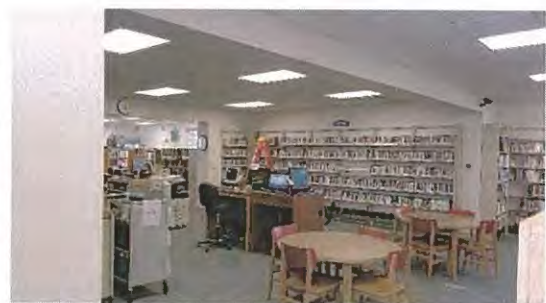
Photograph #12 – Recessed 2'x4' fixture
