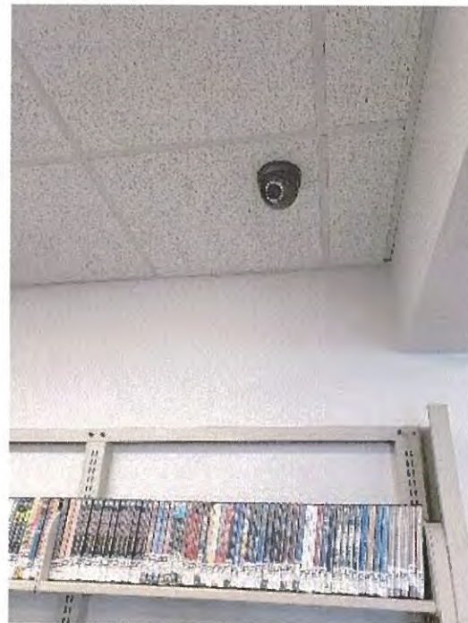
Photograph #17 – Interior Video Surveillance Camera
