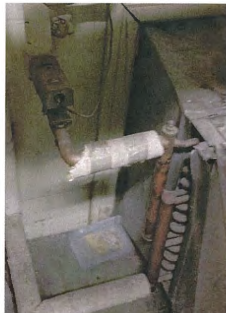
Photograph #4 – Zone #2 Heating Water Coil
