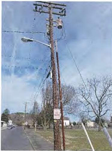
Photograph #9 – Pole Mounted Utility Transformers
