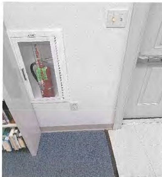
Photograph #13 – Toggle Switches for Control of Lighting
