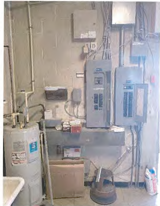
Photograph #11 – Branch Panelboards and wire trough in Boiler Room
