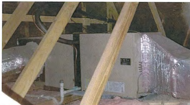
Photograph #5 – Zone #3 Air Handling Unit
