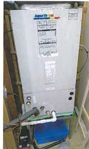
Photograph #2 – Zone #1 Air Handling Unit
