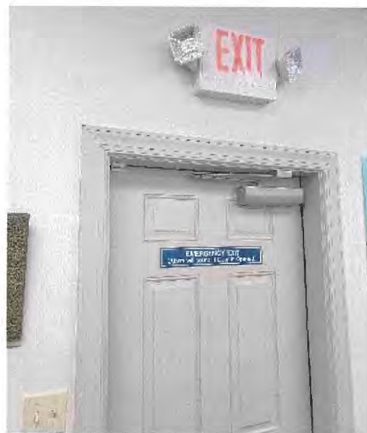
Photograph #14 – Typical Emergency Light Fixture
