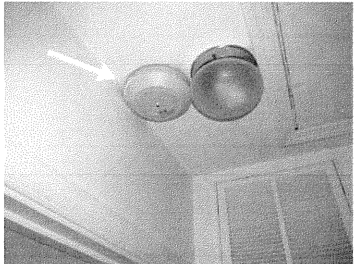
Two smoke detectors would not sound when tested, replace batteries and or units if hard wired.
